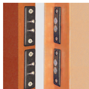
Double electrical contacts between leaf and doorframe
